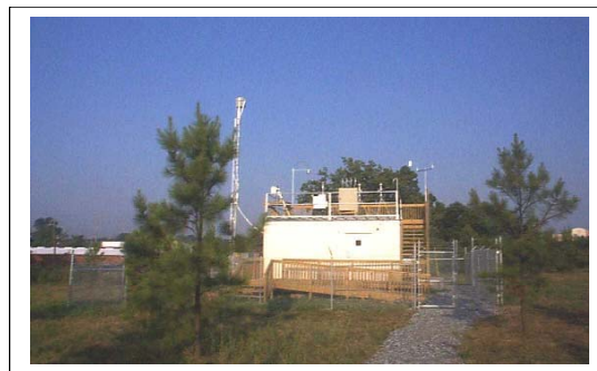
Figure 2. ARIES Central Monitoring Site
